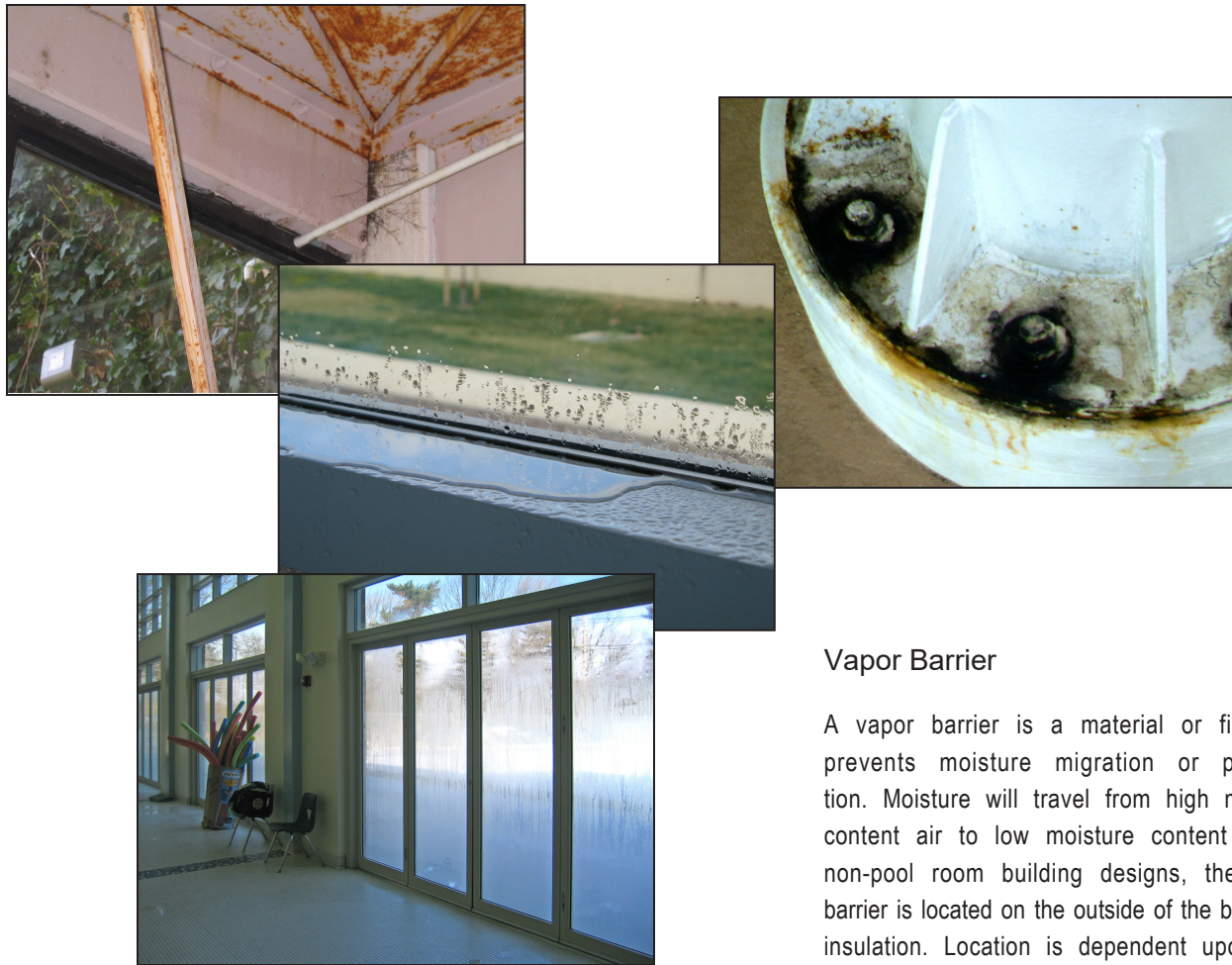
Figure 3. Examples of condensation and poor air distribution
