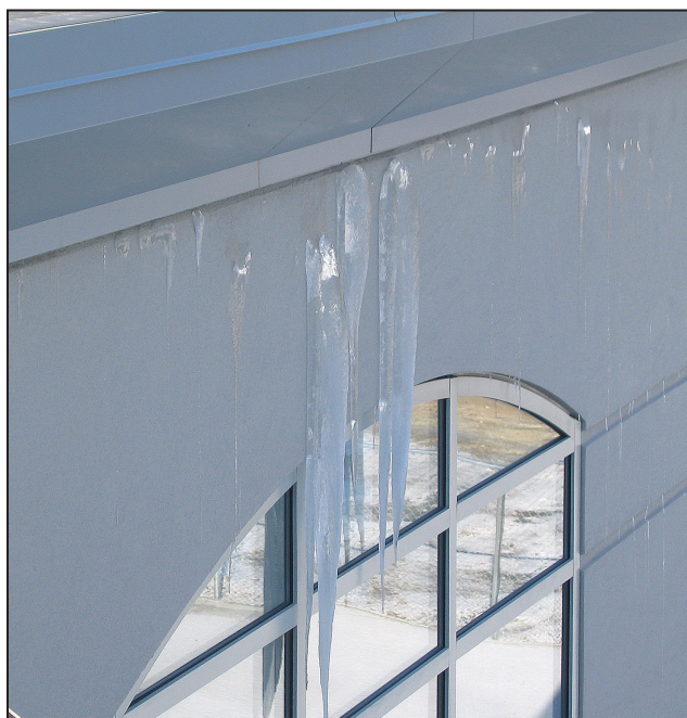
Figure 5. Example of natatorium with improper seals showing moisture migration and icicle formation
