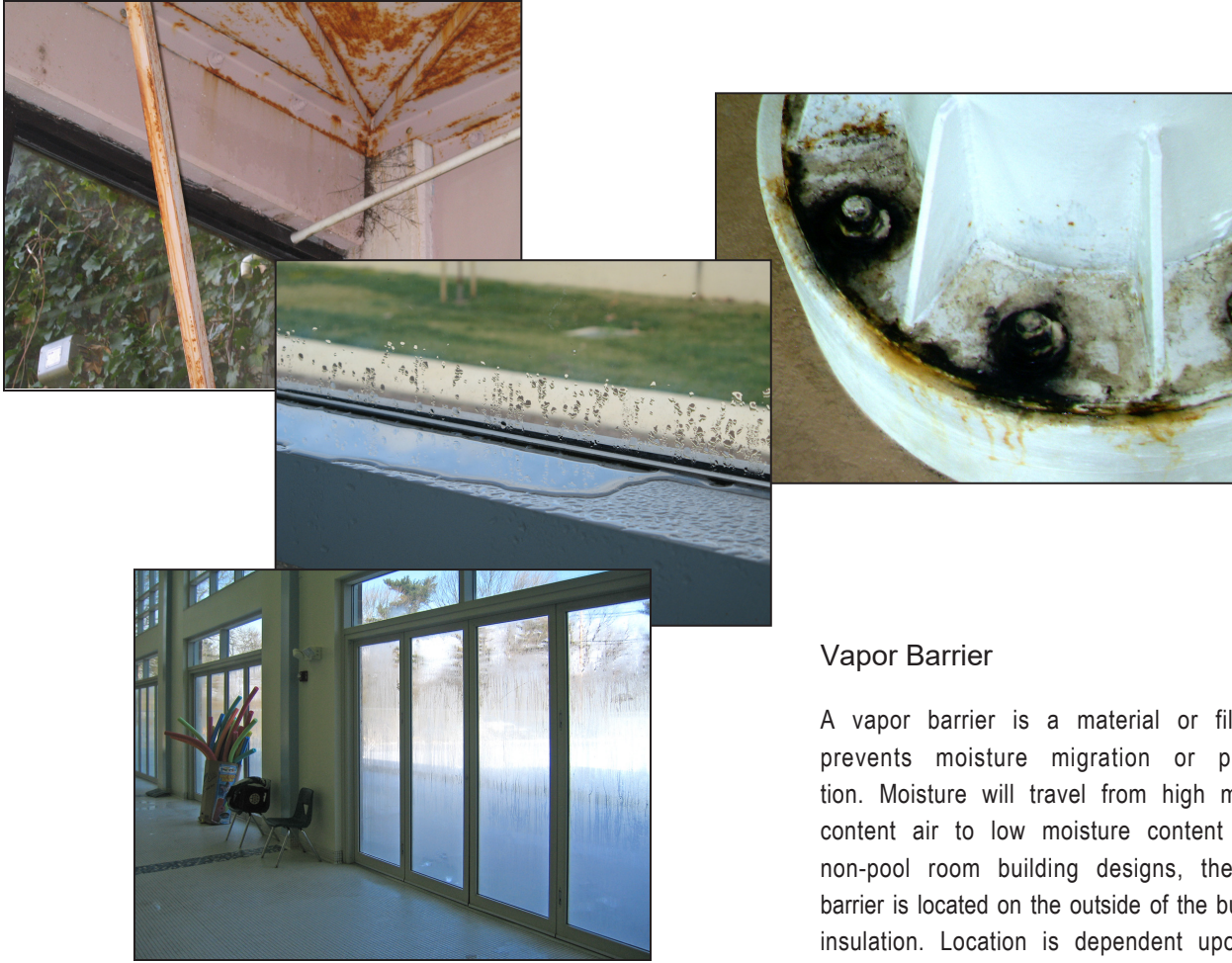
Figure 3. Examples of condensation and poor air distribution
