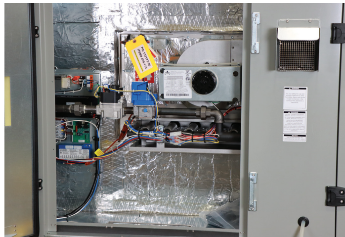
Figure 1 - Detail of Gas Heat Compartment on ExpertAire™ LCQ Series Packaged Unit
