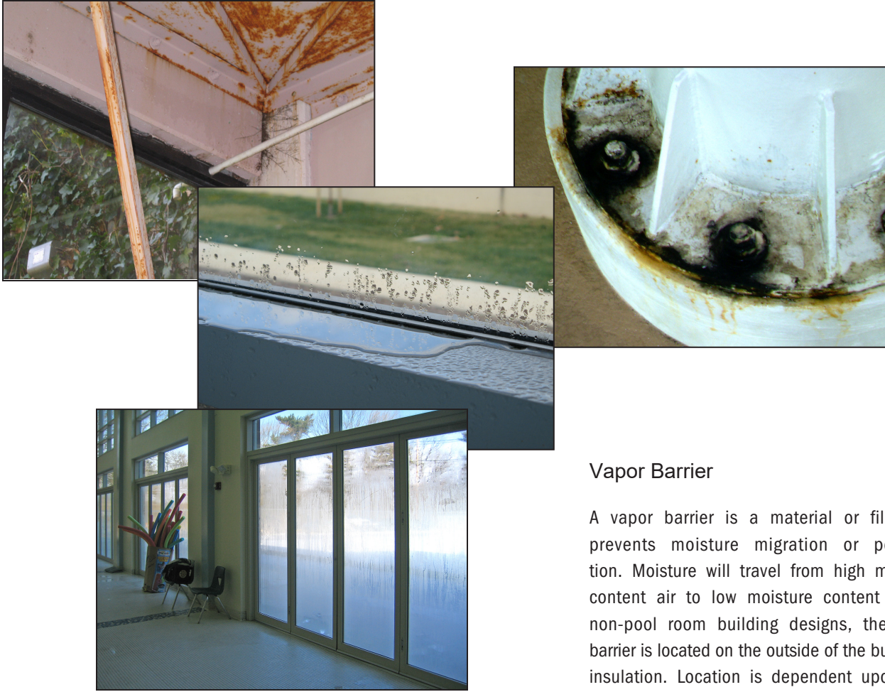
Figure 3. Examples of condensation and poor air distribution
