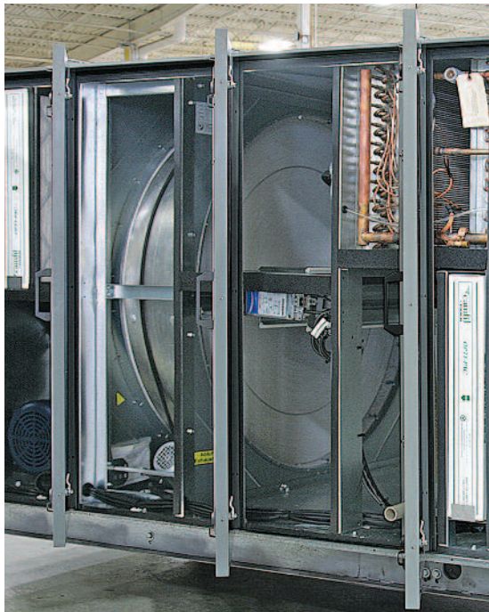
Figure 1 - Enthalpy Wheel Installed in a Desert Aire Aura™ Unit
