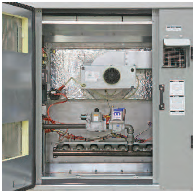
Figure 1 - Detail of Gas Heat Compartment on SelectAire Plus™ Series Unit
