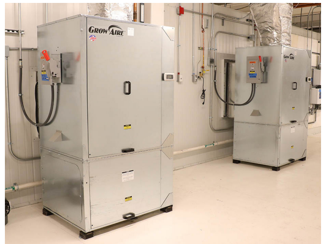
Figure 8 - HVACD Equipment Controlling a Grow Room Environment
