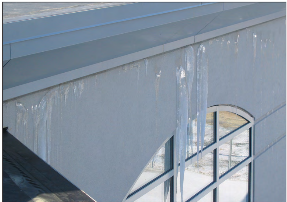
Figure 5. Example of natatorium with improper seals showing moisture migration and icicle formation
