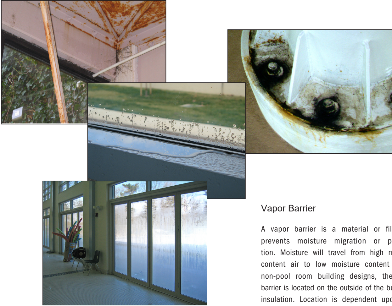
Figure 3. Examples of condensation and poor air distribution
