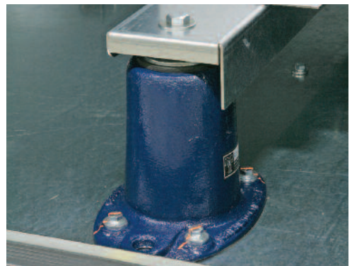
Figure 3 - Spring Isolation Mount Installed on Aura™ Series Unit
