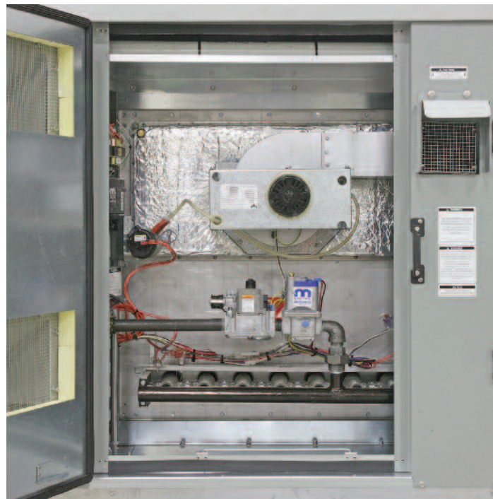
Figure 1 - Detail of Gas Heat Compartment on Aura™ Series Unit
