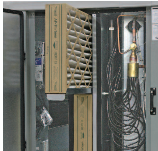
Figure 4 - Filter Rack With MERV 13 Filters Installed.
