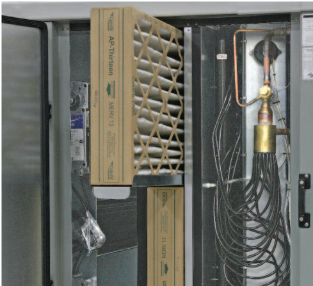
Figure 4 - Filter Rack With MERV 13 Filters Installed.
