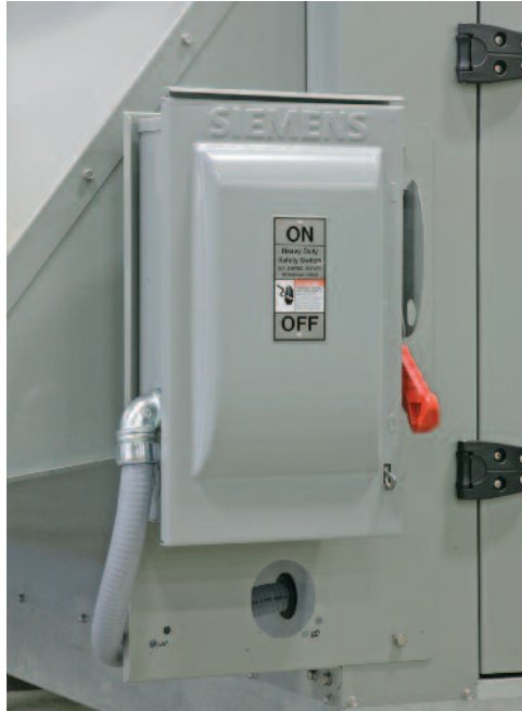
Figure 5 - Disconnect Switch Installed on Aura™ Series Unit
