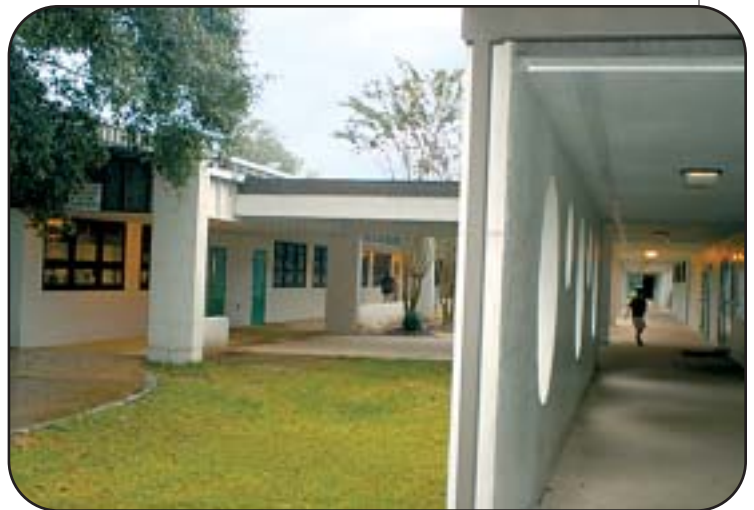
Killearn Lakes Elementary School, which is located in the Leon County, FL school district, opened its doors in 1985. It was one of the district's many schools facing HVAC-related IAQ problems until a dehumidification system was installed in October 2002.
